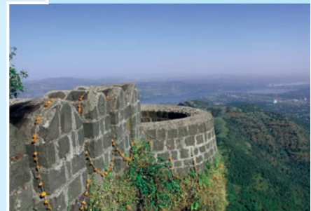
Figure 1.13 : Khadakwasla Dam as seen from Sinhagad
