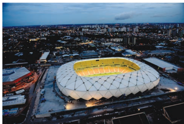
Figure 9.7 : Football Stadium at Manaus
